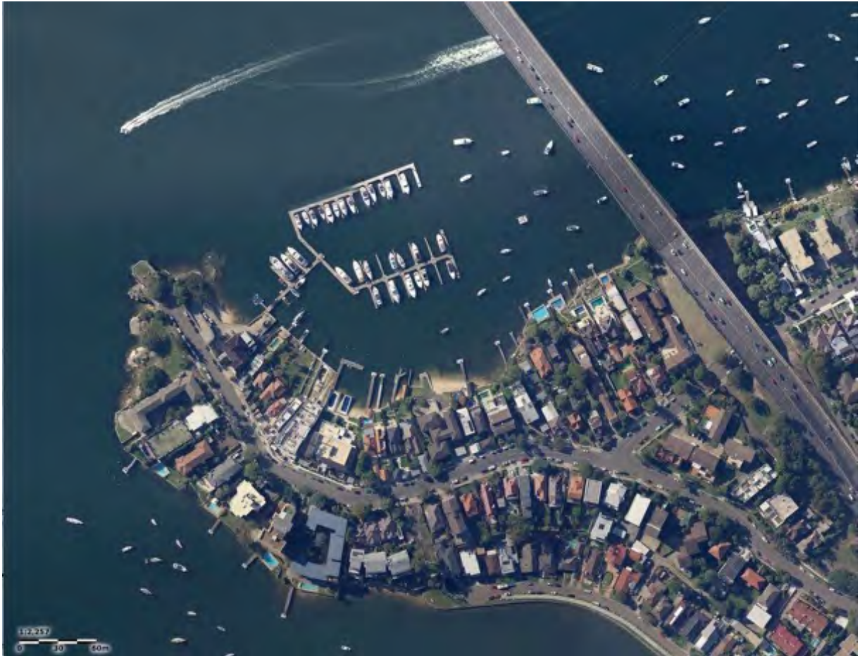
Figure 1: Aerial view of existing Marina in a small embayment west of Gladesville Bridge (NSW SixMap).
