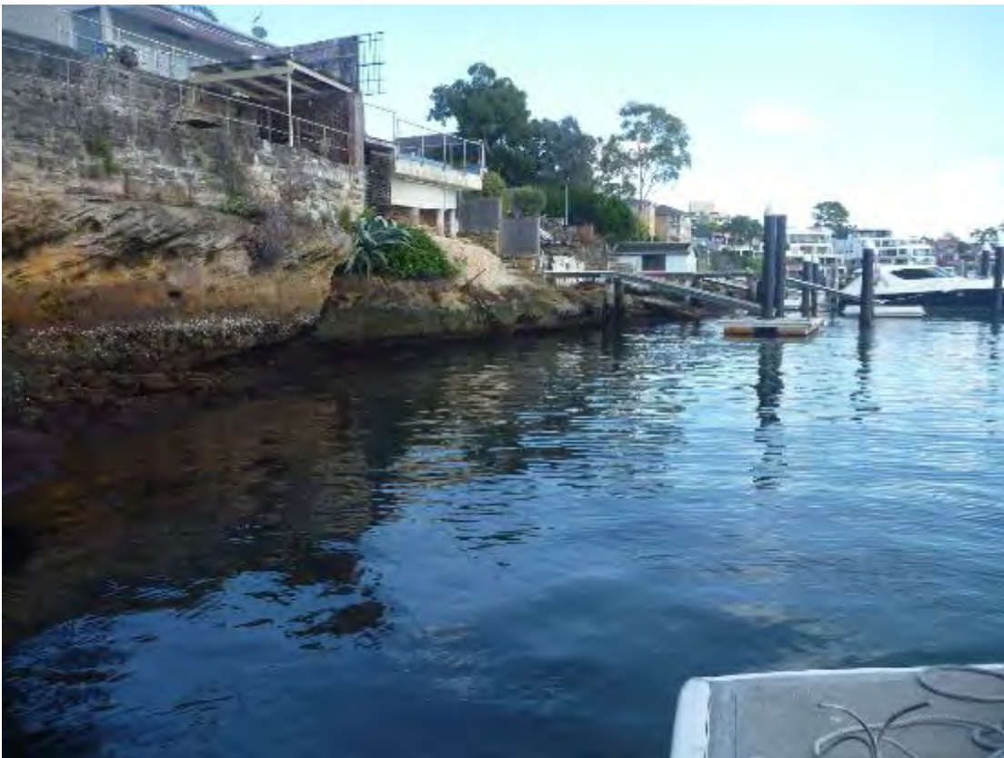
Plate 14: Looking west along rock shoreline from Gladesville Bridge.
