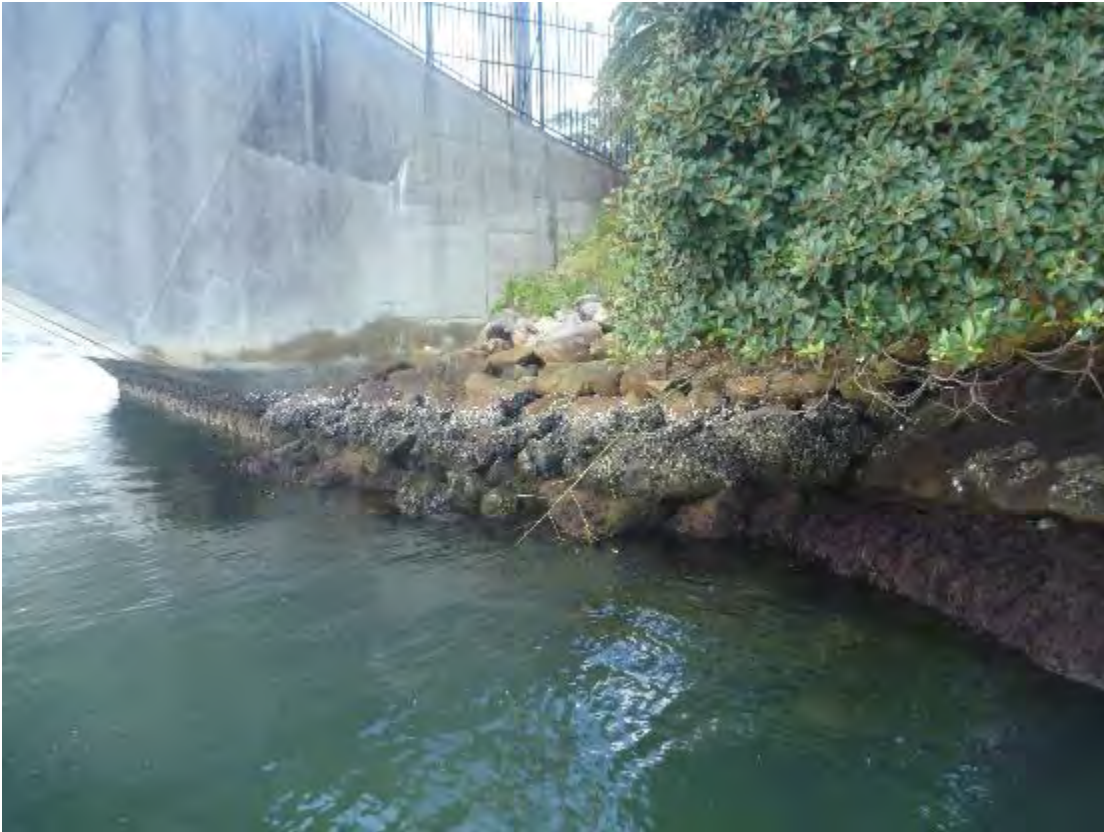
Plate 15: Looking east at the concrete footing for Gladesville Bridge.
