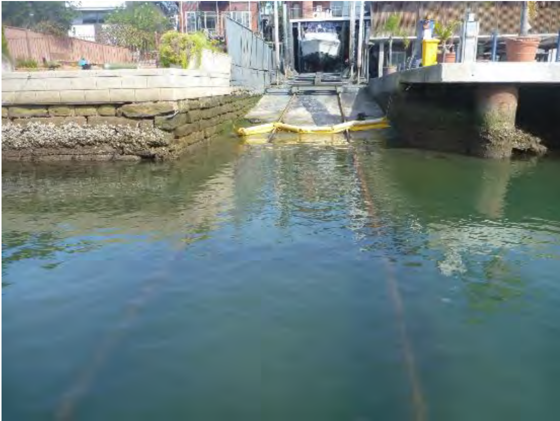
Plate 5: Gladesville Bridge Marina slipway (to be removed under proposal), with beginning of seawall (left hand side) bounding the waterfront residential properties.
