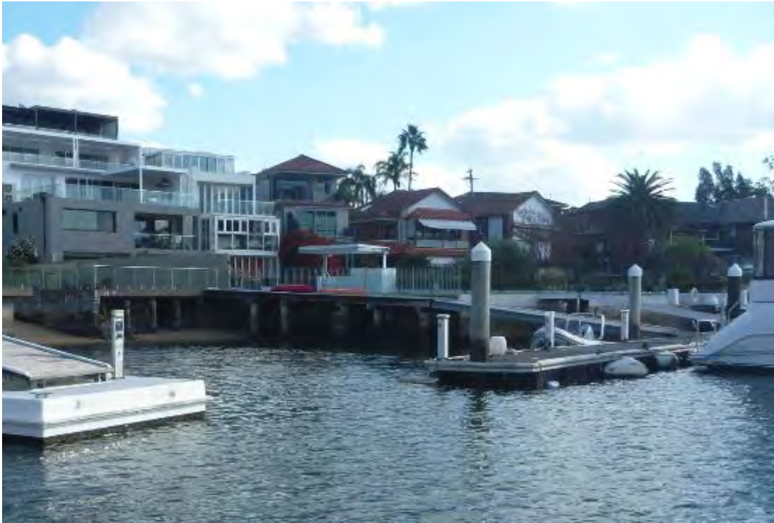
Plate 7: Looking west towards the eastern limits of the seawall in Plate 6.
